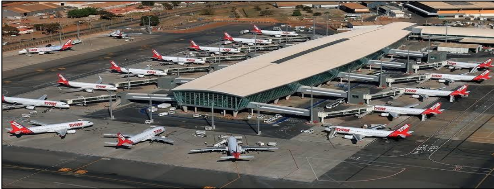
Figure 2 BSB International Airport. Source: Infraero, 2019.
