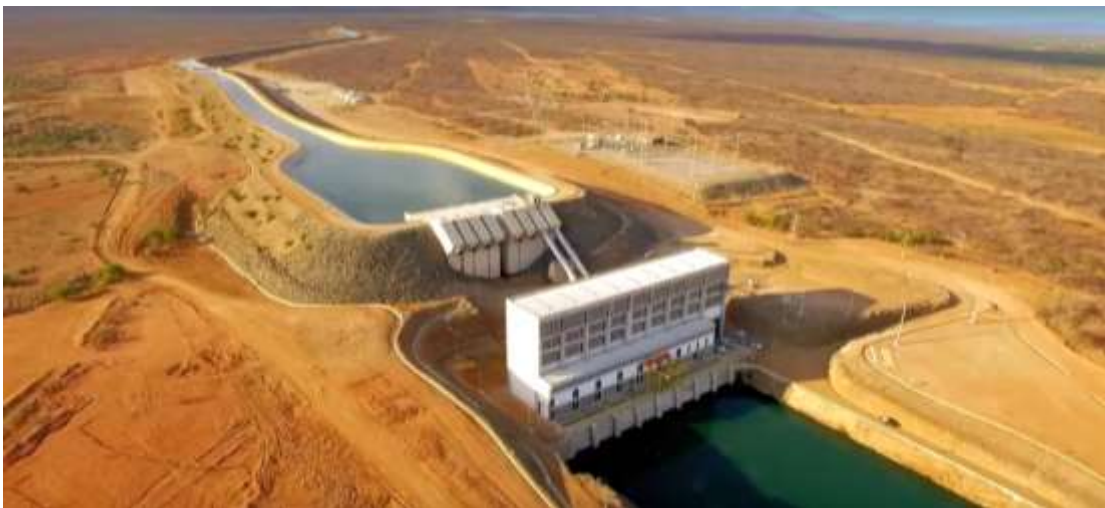
Figure 10 - San Francisco Valley Aqueduct. Source: MIN, 2016
