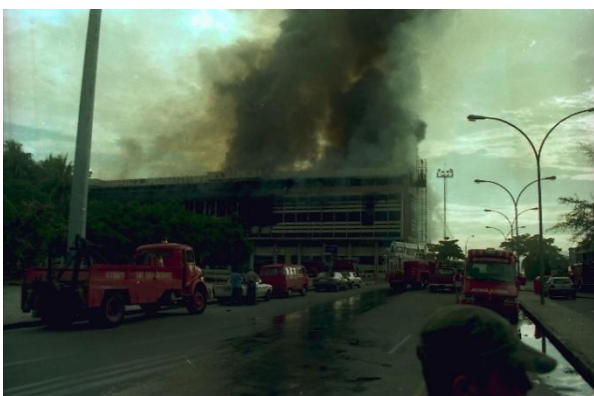
Fig-4: Fire at SDU Source: SDU, 1998 [4]
