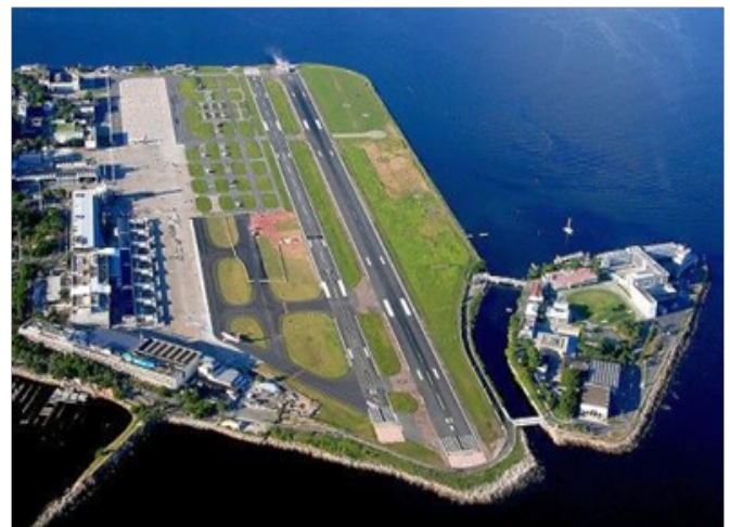
Figure 1: Santos Dumont Airport. Air view. Source: Infraero, 2019.
